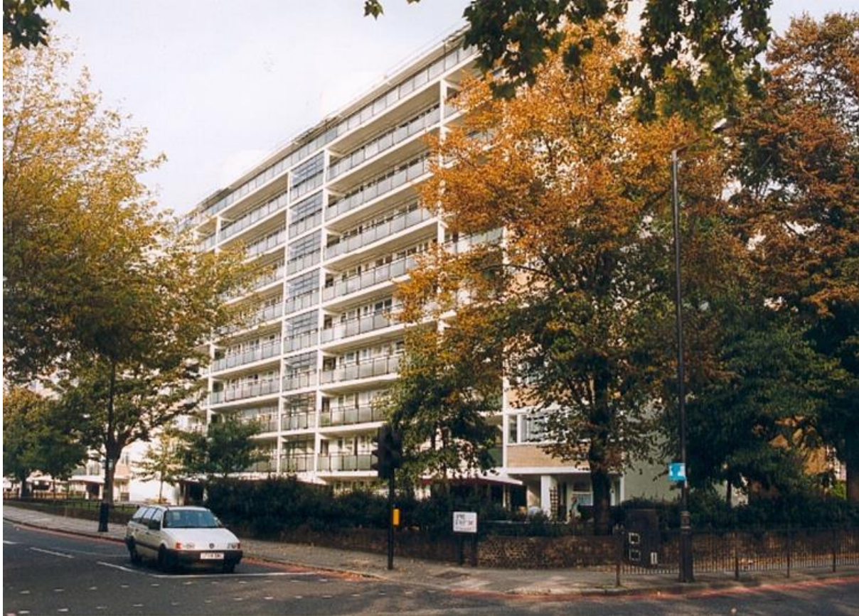
Figure 1. Under S52 of the Water Industry Act 1991 water undertakers are required to maintain the supply of water where domestic premises have been supplied since before 1 st September 1989 – the date of water privatisation. This applies irrespective of altitude or height. So flats on the 10 th floor of this block, which has no water pumps, have a continuing right to receive water under S52.
